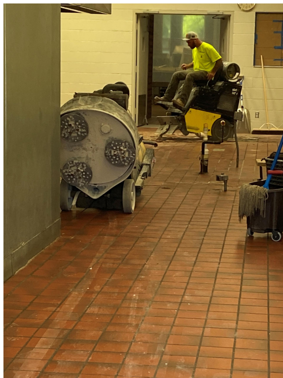
Contractors have begun the removal of the tile.
